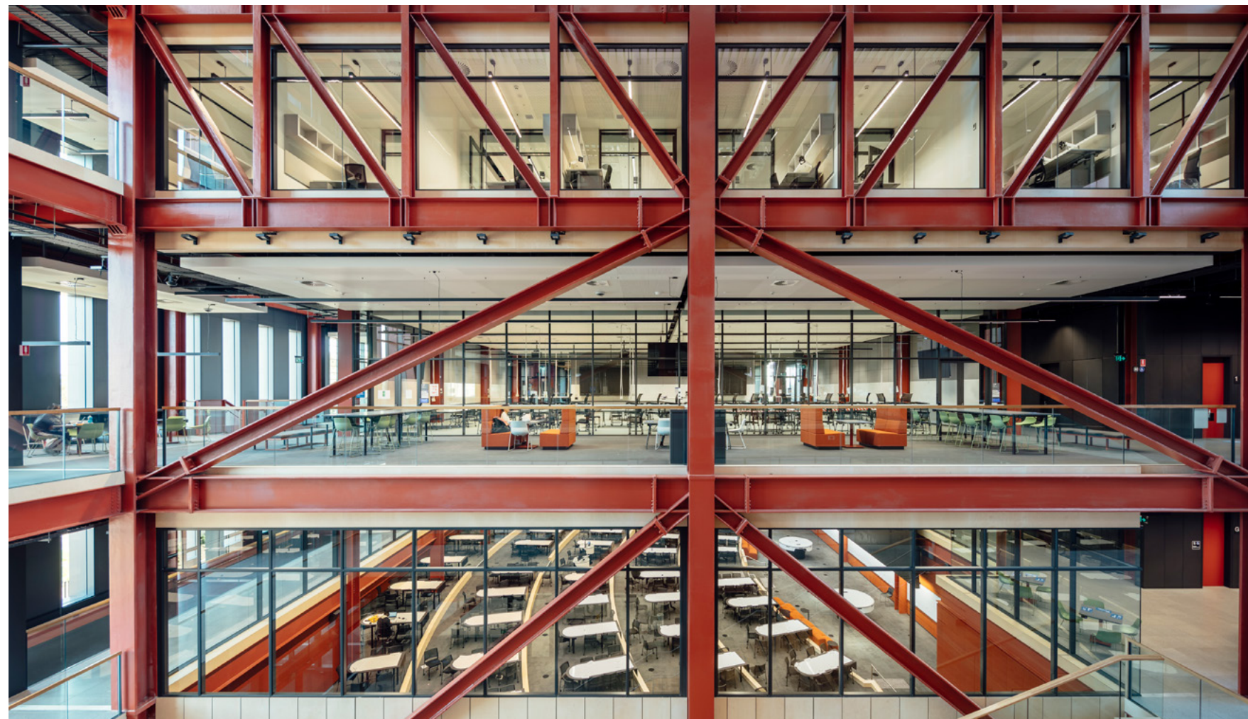
Monash University Woodside Building for Technology and Design , Melbourne, Australia / Architecture: Grimshaw / Lighting design: Arup / Photography: Michael Kai
